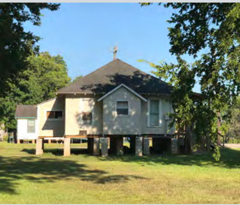
Some homes have been raised temporarily, awaiting final repairs or foundation work until a levee is constructed south of the neighborhood along the Colorado River. Source: ULI Houston.
