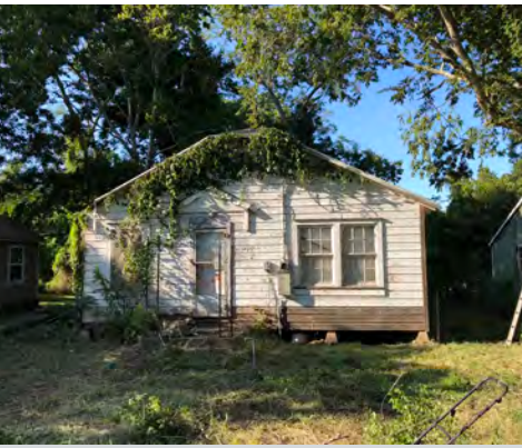
A number of homes in the West End are vacant, awaiting repair following Hurricane Harvey. Source: ULI Houston.
